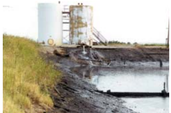
Figure 1. Battery showing produced water discharge to holding pond.
